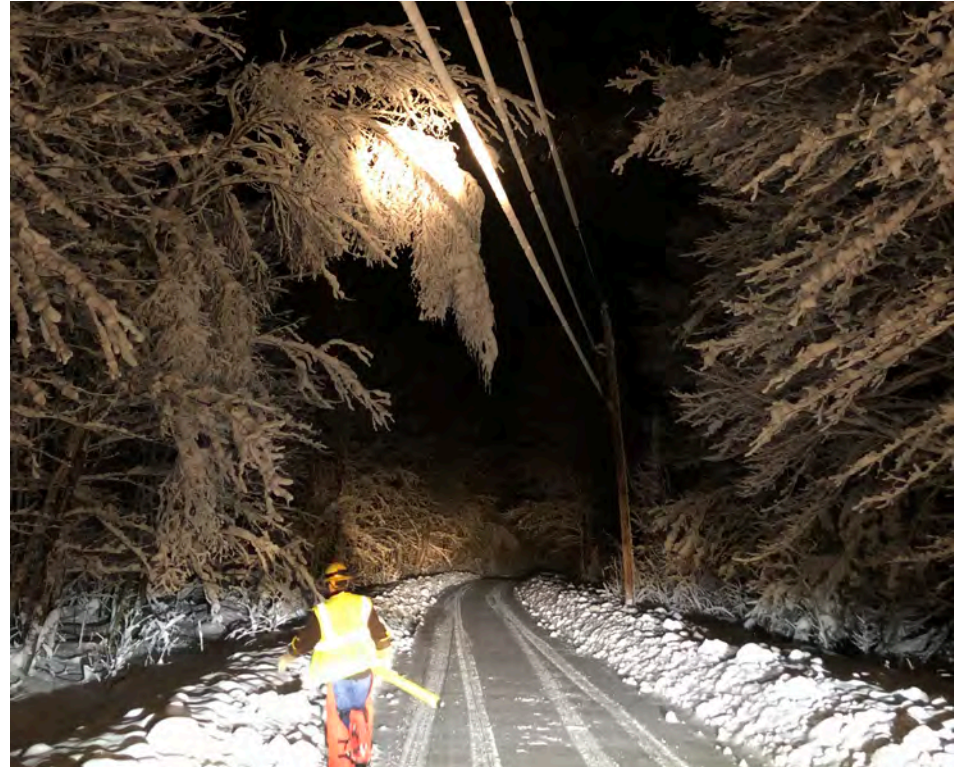
VEC lineworker responding to an outage after Winter Storm Bruce in November/December 2018.
