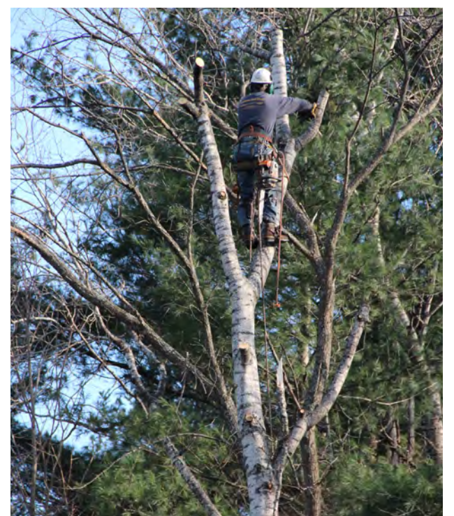
A VEC contractor trims a tree to remove potentially hazardous limbs. This type of work is an integral part of vegetation maintenance.
