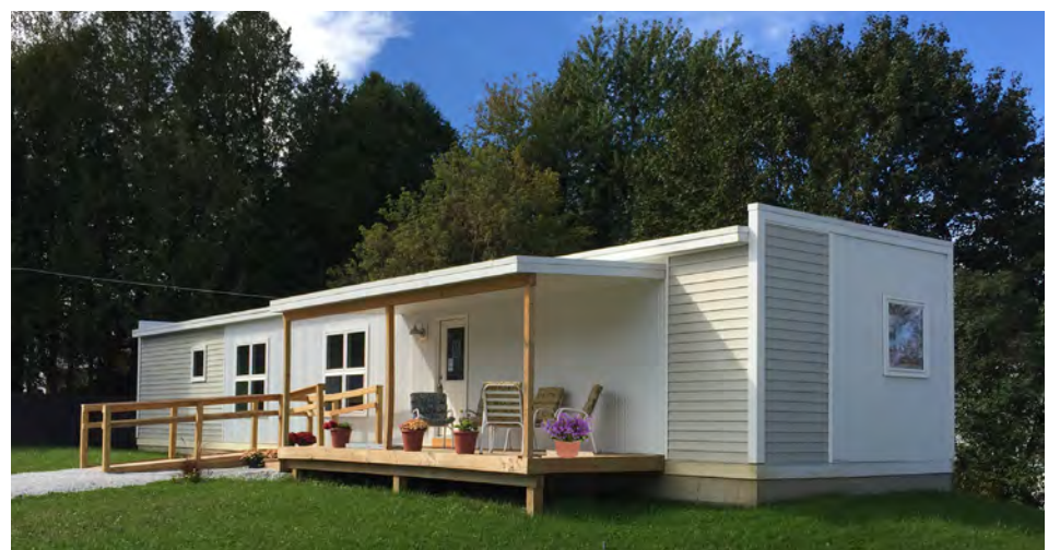
A ZEM home, pictured here, can be a great alternative to traditional manufactured housing, providing greater comfort and more natural light at an affordable cost. Photo credit: Efficiency Vermont
