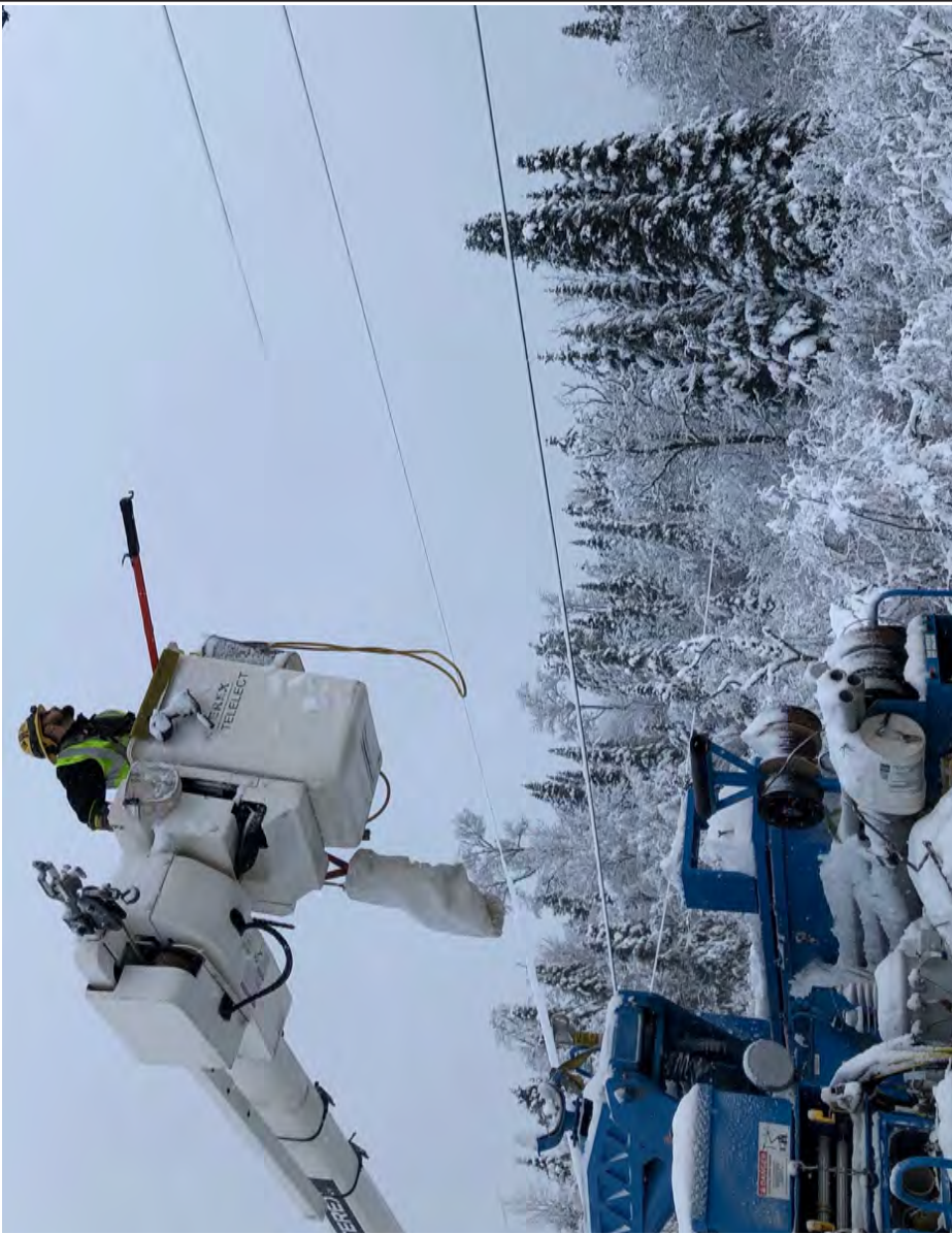
Last November and December, Winter Storm Bruce caused significant outages across VEC territory. Here, VEC line worker Cody Hopkins approaches a line to assess and repair storm damage. In an interview starting on page 1, Chief Operating Officer Peter Rossi discusses how VEC is taking steps to cost-effectively improve VEC's system reliability in the face of increasingly challenging storms.
